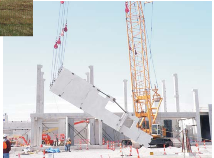
Construction of the Depleted Uranium Hexafluoride Conversion Facility
