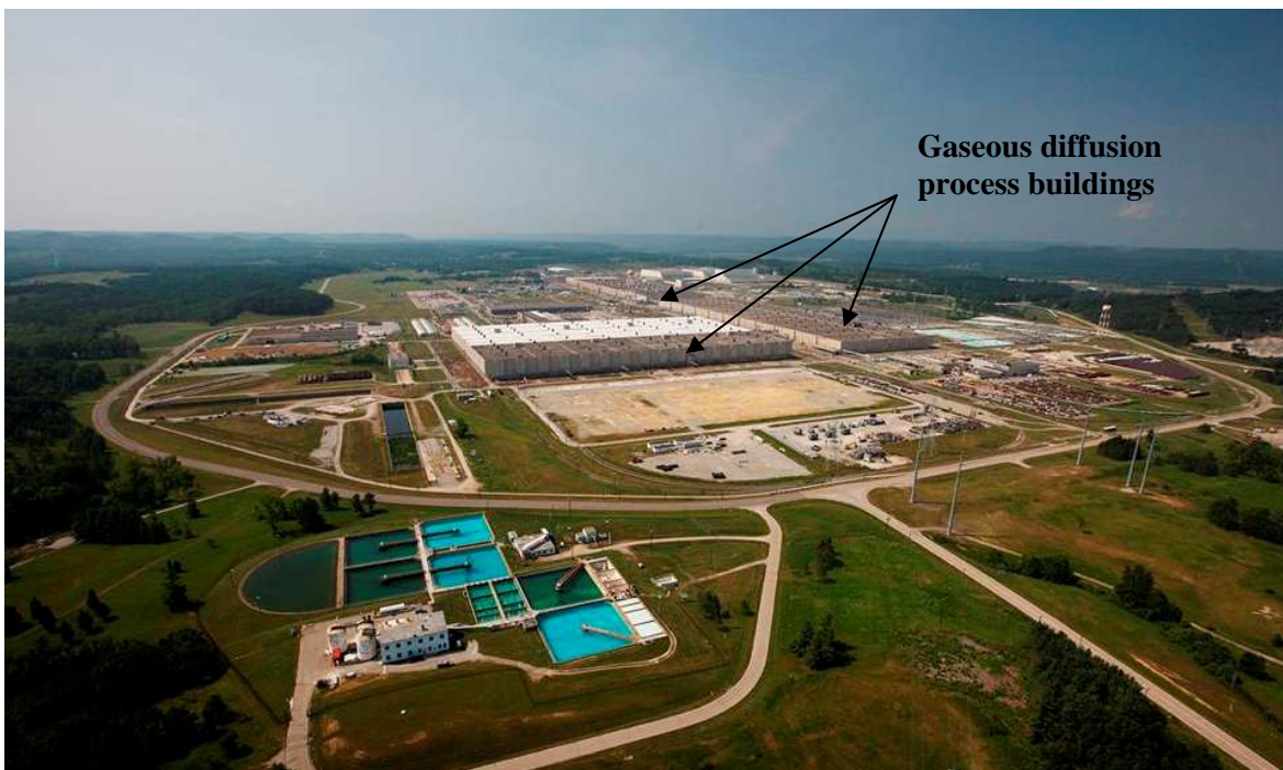
Figure 1.1 The Portsmouth Gaseous Diffusion Plant – 2011.
