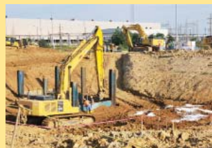
Soil treatment in progress
