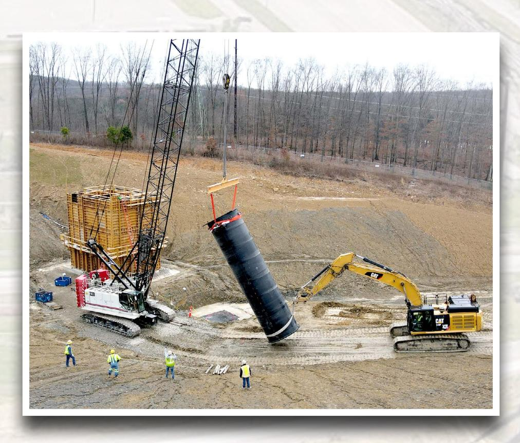
South LTS - 4,200 linear feet of piping for the monitoring trench, 5 valve houses, 32' deep lift station (pictured) installed.
