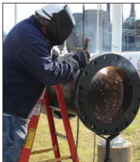
Chuck Scott, Geiger Brothers, welds a flange section to the steam pipe.
