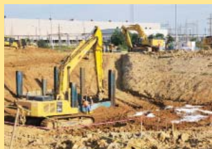
Soil treatment in progress
