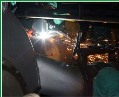
Compressor detached from interconnecting piping using a plasma torch.
