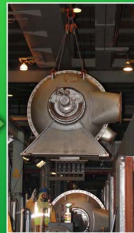
Compressor is lifted from the cell housing
