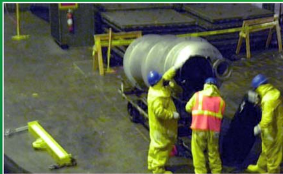
Metal plates are welded to secure the openings.
