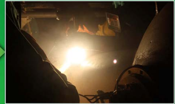
Converter detached from the interconnecting piping using a plasma torch.
