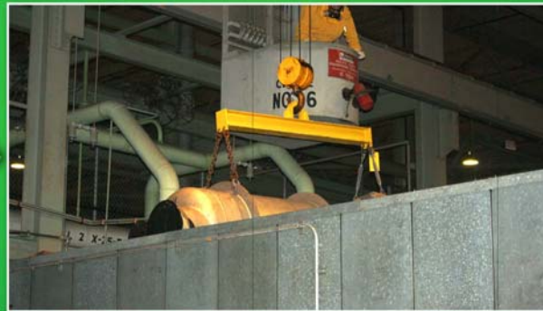
Converter is raised from the cell using the crane.
