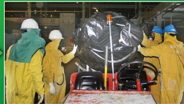
Converter is wrapped in plastic for contamination control and moved to the Operating floor to await shipment to the Nevada National Security Site (NNSS) for disposal.
