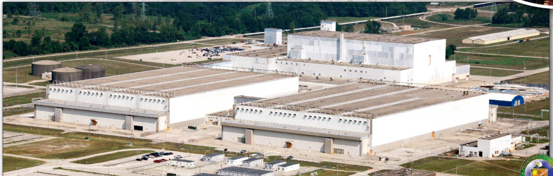
2011 Aerial view looking northwest
