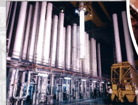
Original GCEP machines being put into place
