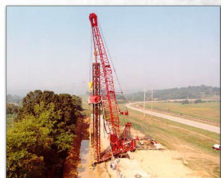
1994 Subsurface barrier installed
