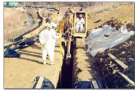
1991 Trench system built to protect Little Beaver Creek
