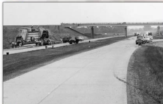
1954 Construction of access road on US Route 23
