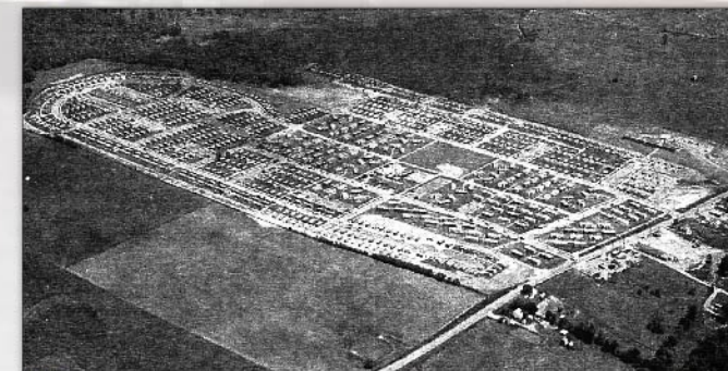
1954 Worker camp aerial view
