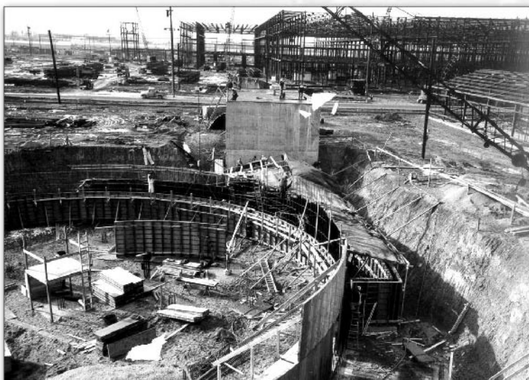
1953 Plant Control Facility X-300 construction
