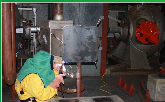
Process gas cooler being removed from the Freon and process gas systems.
