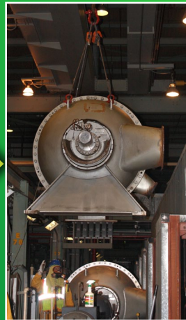
Compressor is lifted from the cell housing
