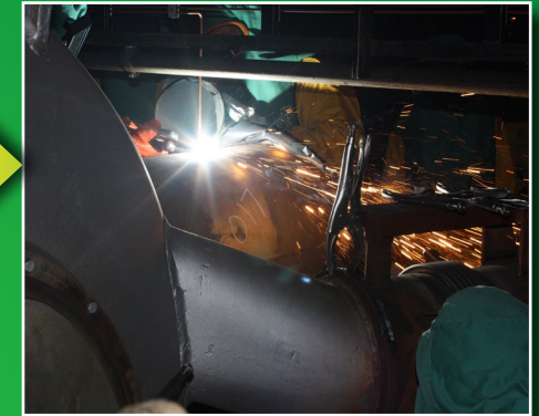
Compressor detached from inter-connecting piping using a carbon arc torch.
