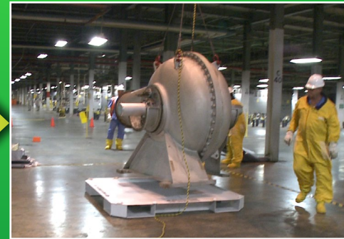
The compressor is lowered to the operating floor.
