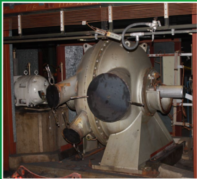
Metal plates are welded to secure the openings.
